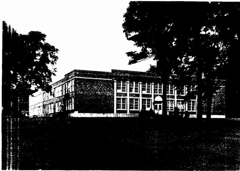
North Plainfield High School, new and modern in design and construction.
