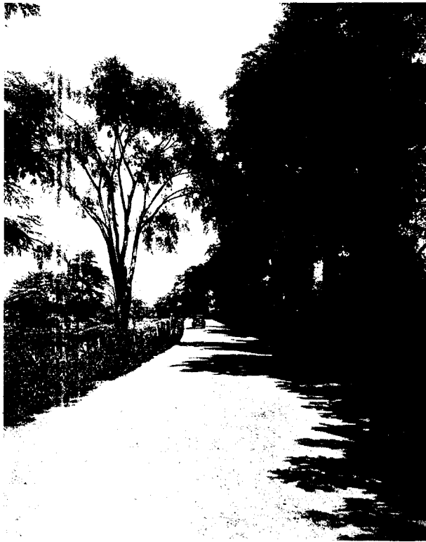
Green Brook Road in N. Plainfield Twp. after retreading with small crushed stone—such as is furnished by the Bound Brook Crushed Stone Co., Wilson Quarry Co., Smalley Stone Co., and Morris County Crushed Stone Co.
