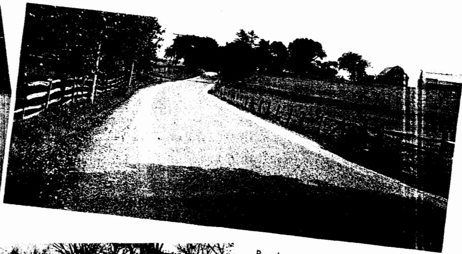
Road at Peapack top-dressed—with slag supplied by the Duquesne Slag Products Co., Philadelphia, Pa.
