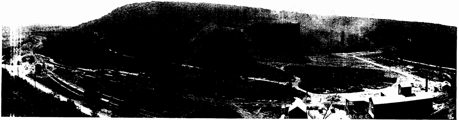
Bound Brook Crushed Stone Co. quarry and plant in action.
